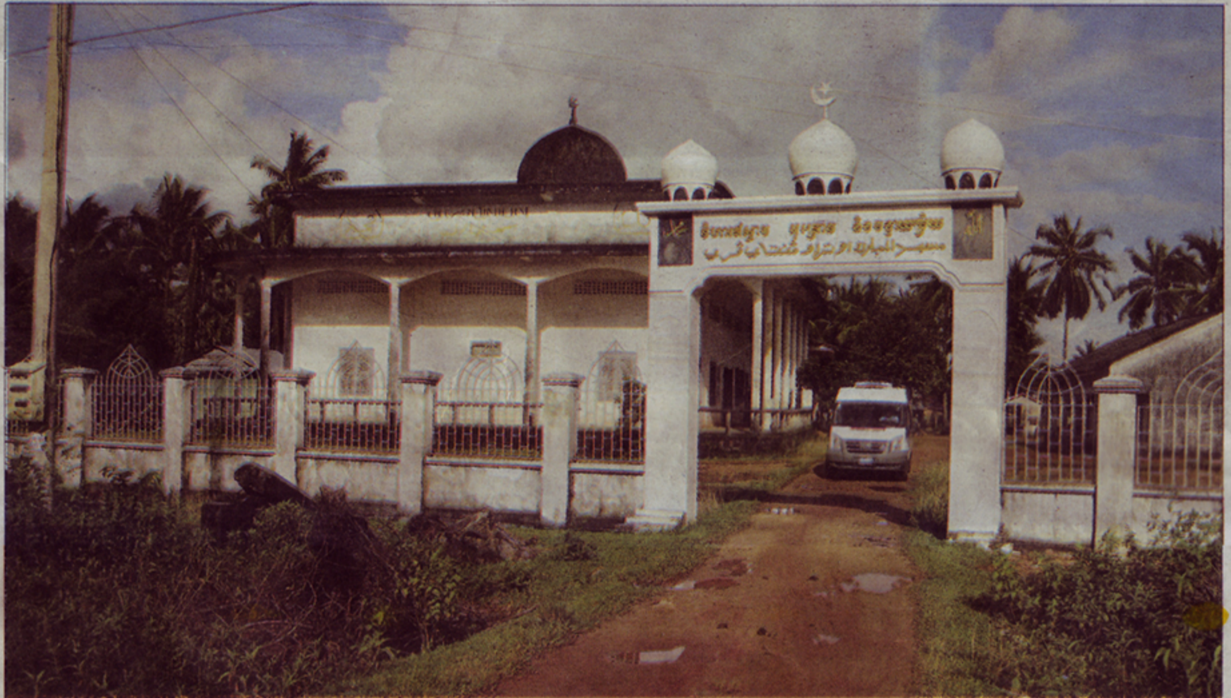
The 50-year-old Al Mubarak mosque in O-Trav village, Andaung commune. The roof sinks when it rains, according to a religious leader. DOCUMENTATION CENTER OF CAMBODIA
